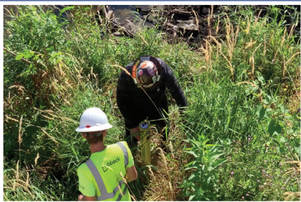
Locate cable on shore
